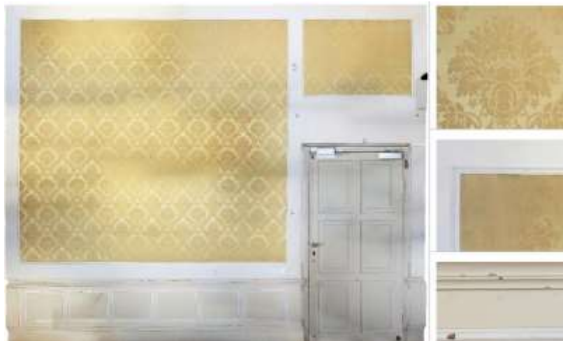
Figure 8. The final orthoimage generated from the integration of point clouds from TLS and image matching. Zooms presents selected elements of the materials
