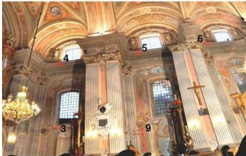
Figure 9. The example of the location of the measuring points in the nave (points 4 - 5) and of the bark gauges (points 3 and 9) [45].
