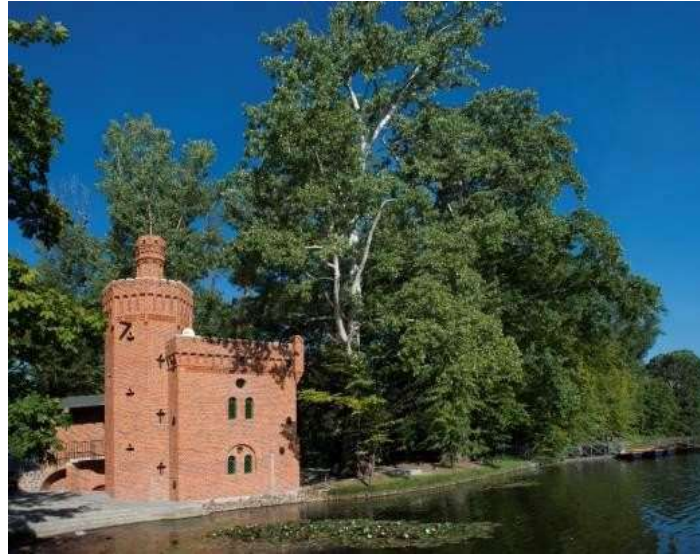
Figure 2. View of the pumping station from the side of Wilanow Lake (photo: W. Holnicki)
