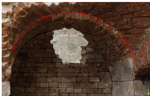
Figure. 3 Stereo measurement of the arch contour and determination of point coordinates
