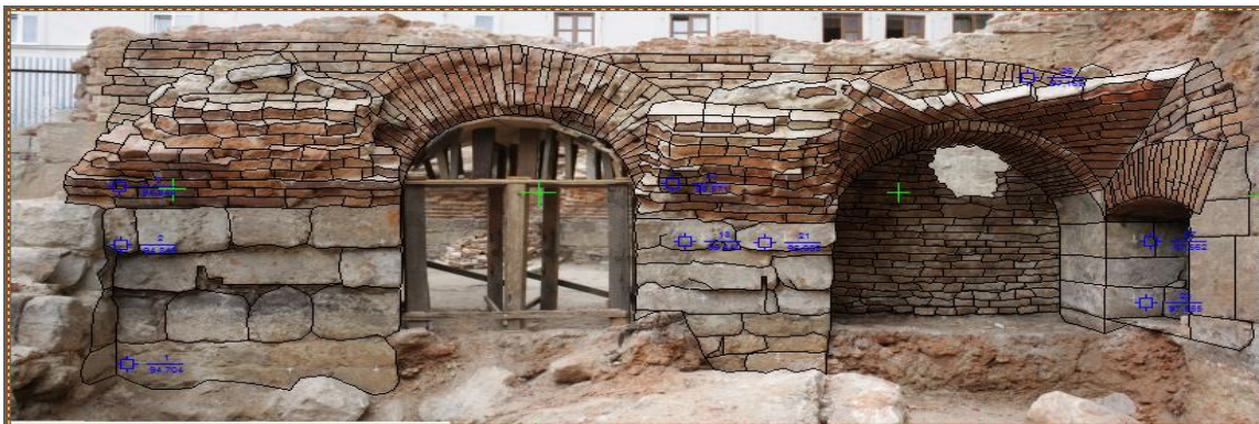
Figure. 2 The vector drawing integrated with the orthoimage
