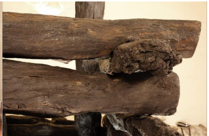
Figure 2. Precise photo of the structure
